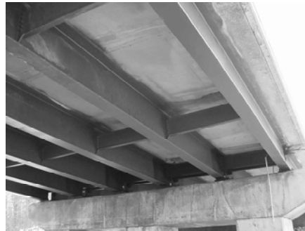
Figure 11 I-189 Spear St. overpass bridge with diaphragms
